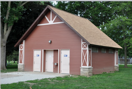
Perkins Park Restrooms located near the shelterhouse.
