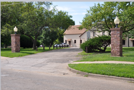
Perkins Park Shelter House from Dill Street Entrance
